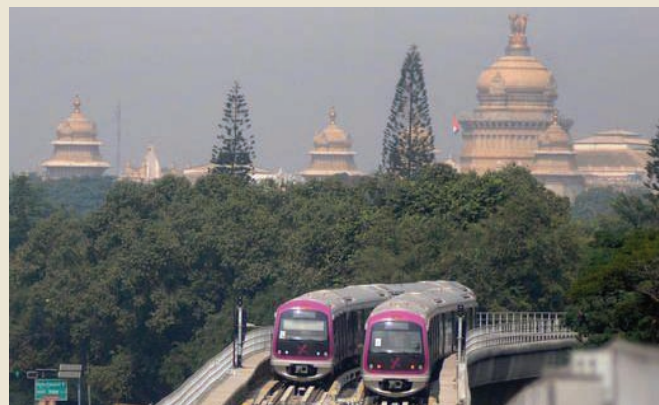
Metro near M.G. Road, Bengaluru
